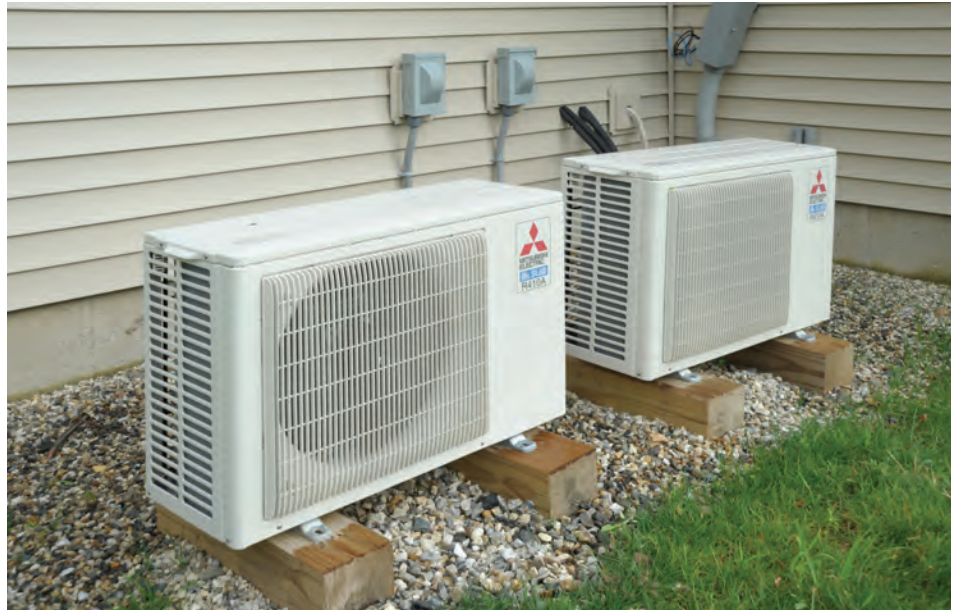
Mitsubishi dual-stage heat pumps produce 92 percent of their capacity at 5°F (minus 15°C) and keep producing heat down to minus 13°F (minus 25°C).
